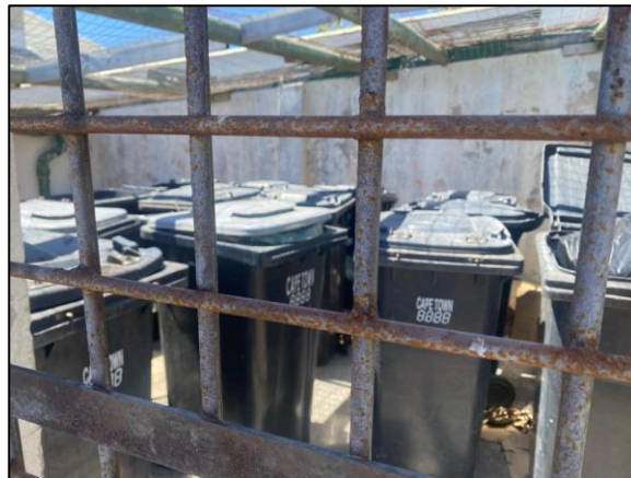
Figure 8. Waste storage area at Signal School.
